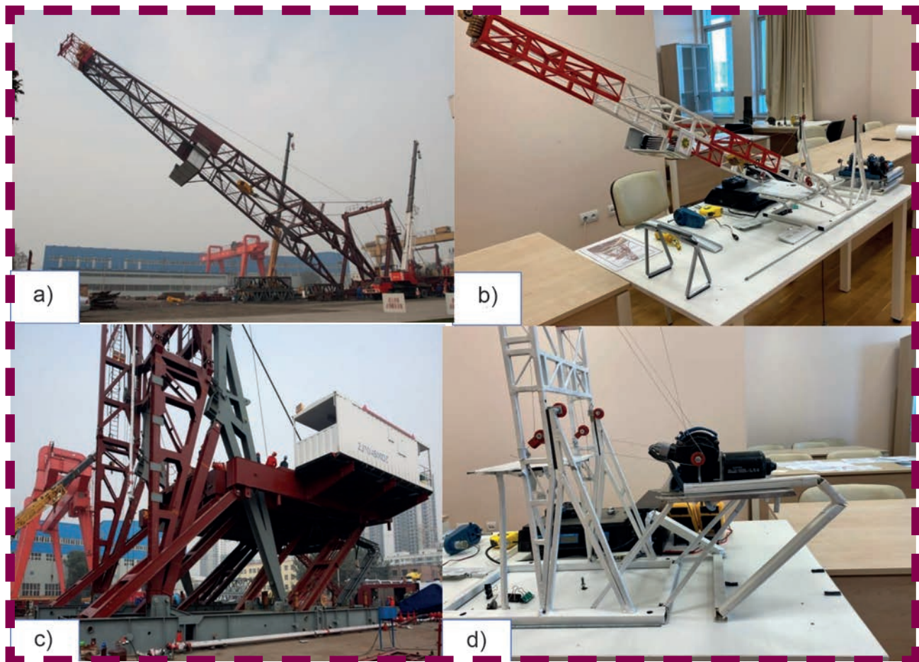
Picture 2- Some moments of rig installation: a) and b) the moment of the mast lifting. c) and d) the moment of lifting the drilling platform
